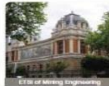
ETSI of Mining Engineering
